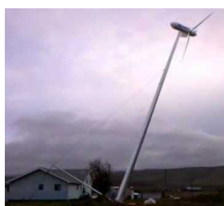
Figure 2.4 Failed foundation resulting in a tilted wind turbine tower
